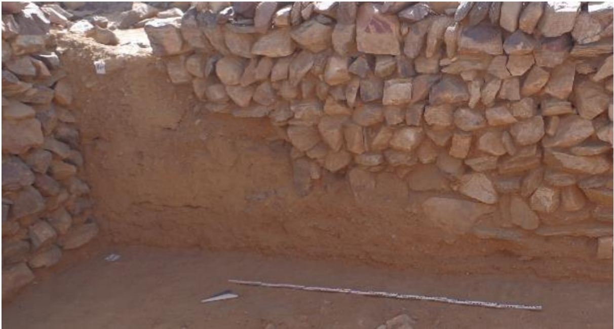
Figure 6: Pisé repairs at the eastern wall at trench 08
